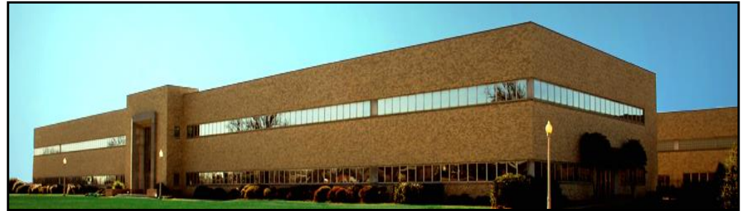
DataChambers Data Center Facility
